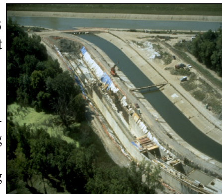
Construction of Detroit's Hubbell-Southfield Combined Sewer Overflow Retention Treatment Basin
