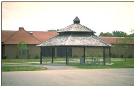
Dearborn Heights Combined Sewer Overflow Retention Treatment Basin
