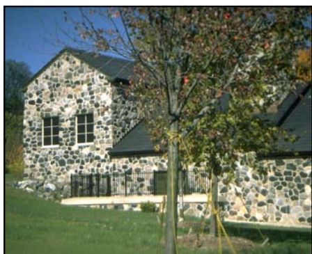
Birmingham Combined Sewer Overflow Retention Treatment Basin
