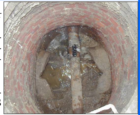
Illicit Connection: Broken sanitary sewer line within a storm sewer manhole
