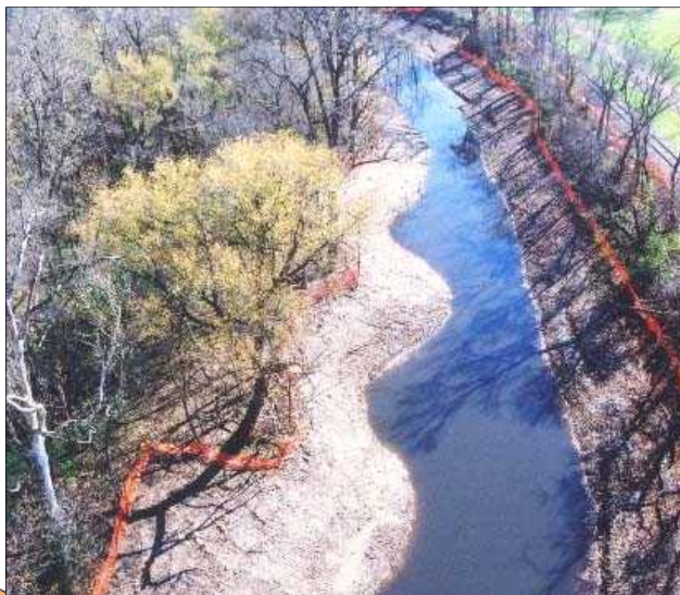
Rouge Oxbow Restoration at Greenfield Village, Main Rouge River
