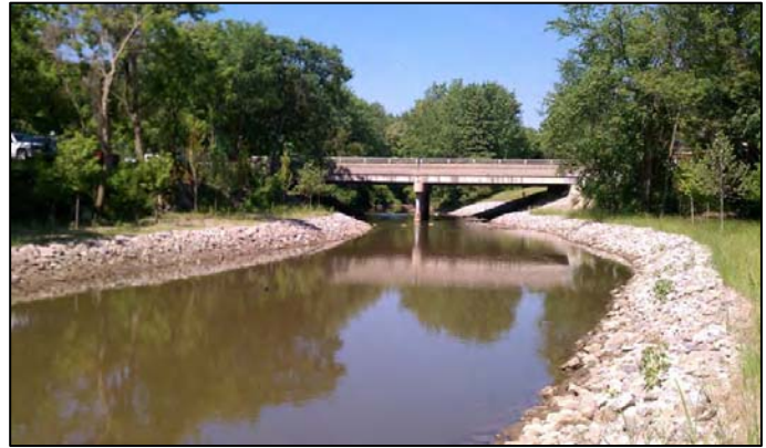
Lower Rouge at Wayne Road after Dam Removal and Stream Restoration
