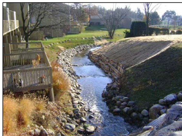
Stream Restoration, Randolph Street Intercounty Drain, Middle Rouge River
