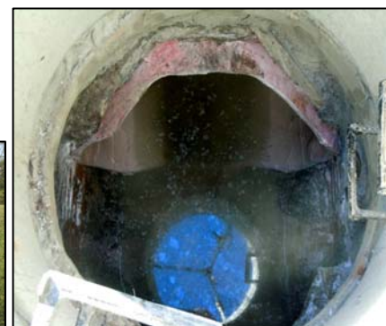
Sewer Lining for SSO Control
